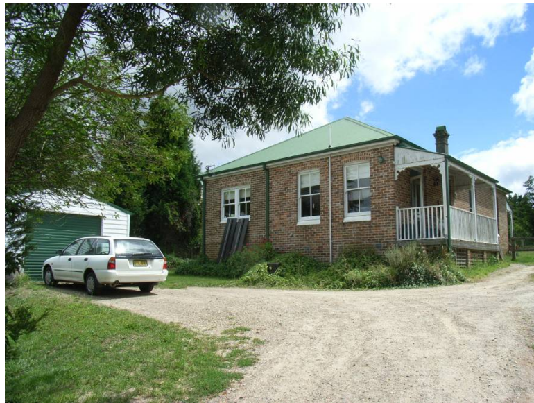
Photograph 5 - Existing Workers Cottage on site
